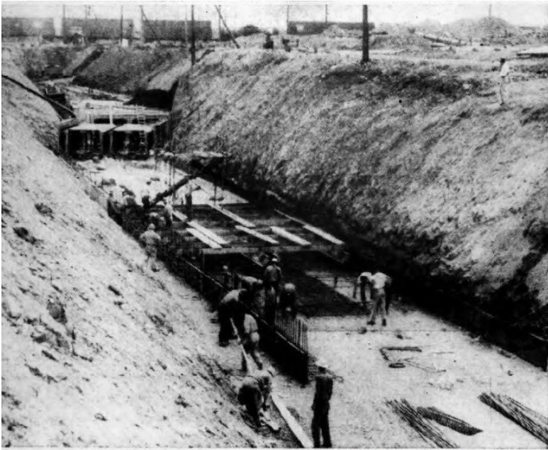
The 1957 massive storm sewer negatively impacted the course directly and indirectly
