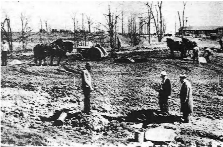
Construction of the Sheridan Golf Course in 1932
