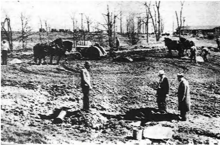
Construction of the Sheridan Golf Course in 1932
